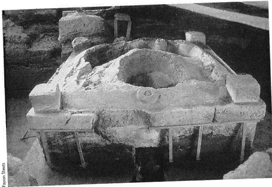
Figure 6-8 Structure 9, looking south. The bajareque adobe dome was destroyed in two areas by lava bombs. The dome originally was protected by a thatch roof supported on roof beams resting on the four short adobe columns.
