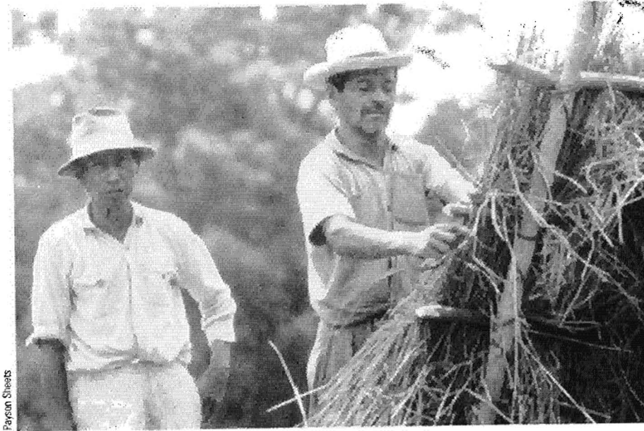
Figure 2-2 The father of the family placing thatch on a small field house in the cornfield, to be used as shelter in a sudden rainstorm. The grass thatch is tied to the roofing supports. Good thatch roofing was essential to the adobe architecture of Ceren. The other man (left) is a friend who helped gather the wooden supports and thatching material. The two unrelated men are good friends and often help each other with various agricultural activities.
