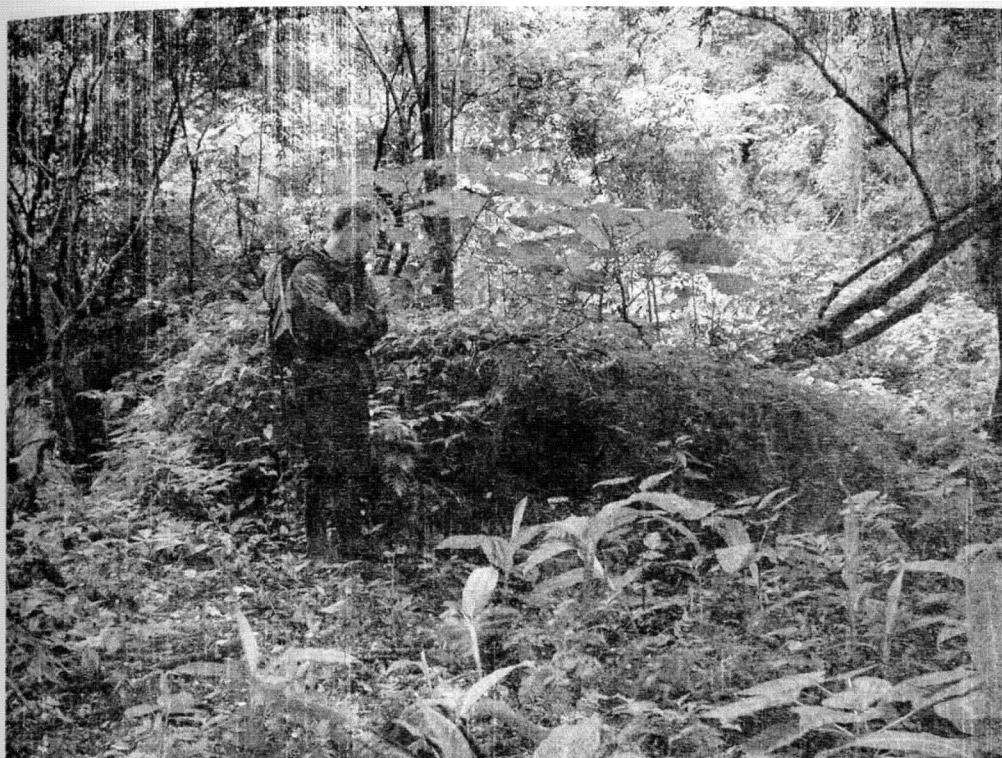
Fig. 5 Horno 2, the main opening is just to the right of the author in this picture.
